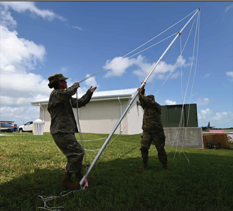
BOTTOM: 920th Communication Flight Airmen setup a High Frequency antenna during an exercise in early October. The HF Frequency antenna is used to transmit between 3 - 30 hertz and can transmit up to 6,000 miles line of sight.
