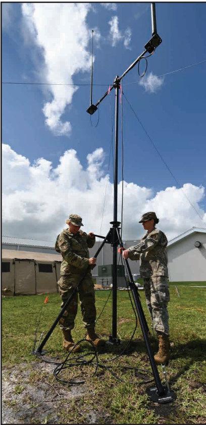
RIGHT: 920th Communication Flight Airmen raise an antenna mast with two line of sight antennas which are used to pass voice and data information between aircraft and members on the ground during an exercise in early October.
